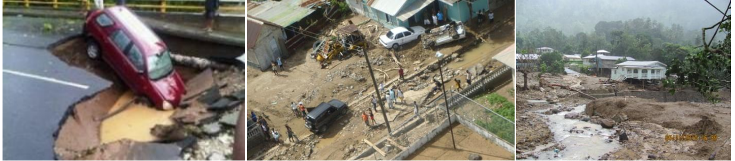
The storm caused floods, road collapses, landslides and infrastructure damage . [© NEMO, Ministry of Finance, Economic Affairs, Planning & Social Security, MapAction]
