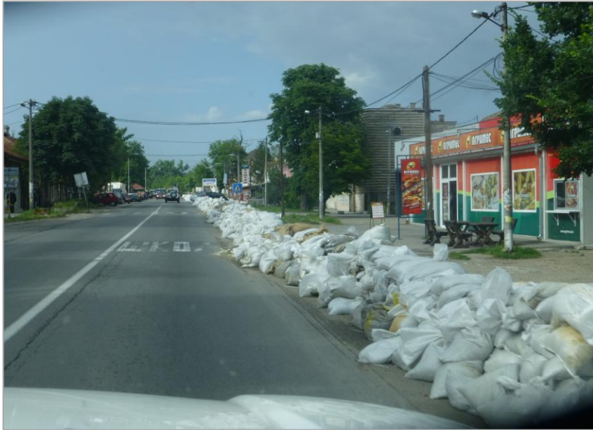
1-2m of sandbagging along the main road between Belgrade and Obrenovac [© Alan Mills MapAction]
